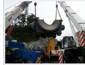
Seating the Exist LP Lower Casing
